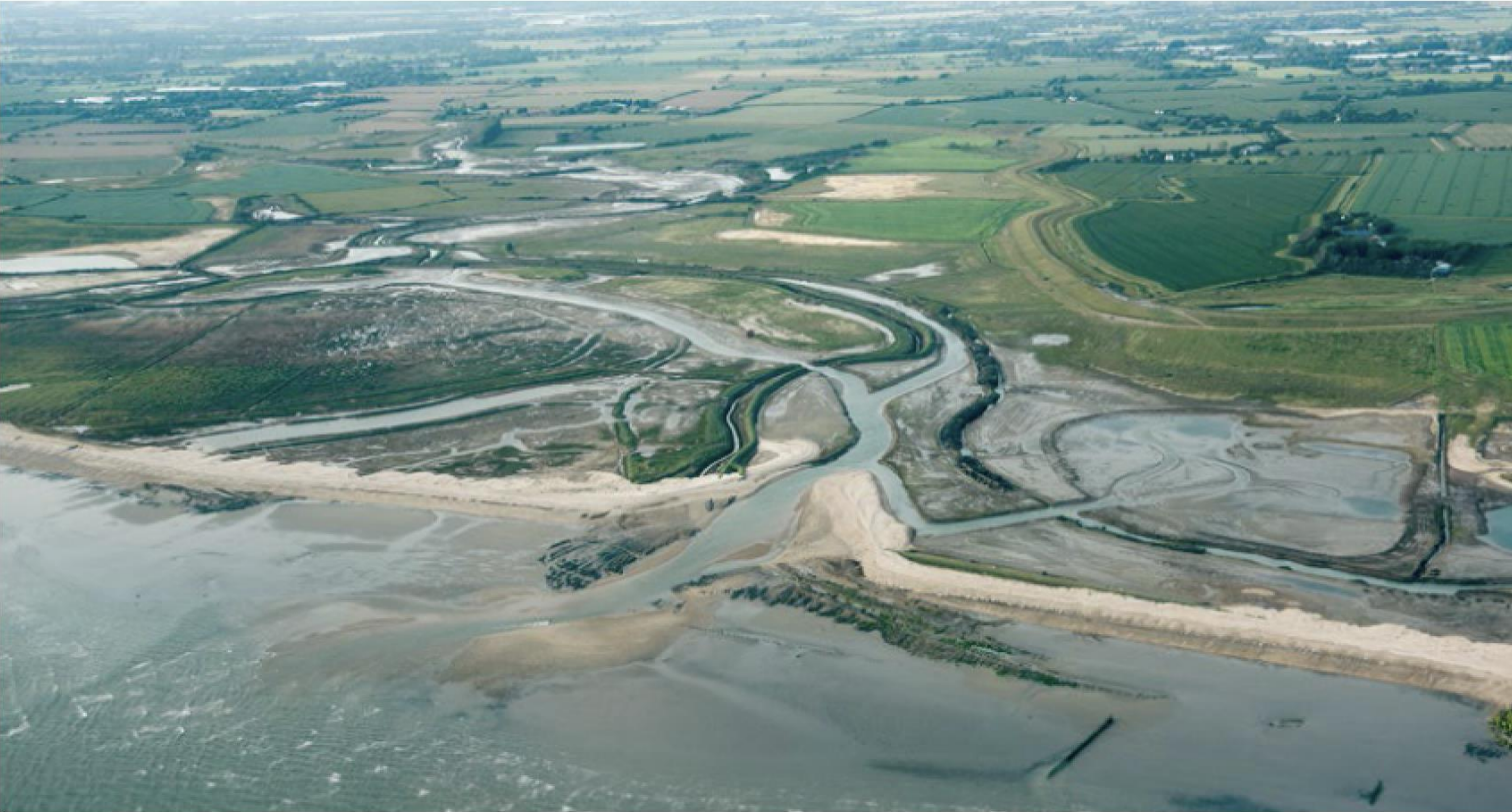
Aerial view of managed realignment at low tide - Photo credit: UK Environment Agency
